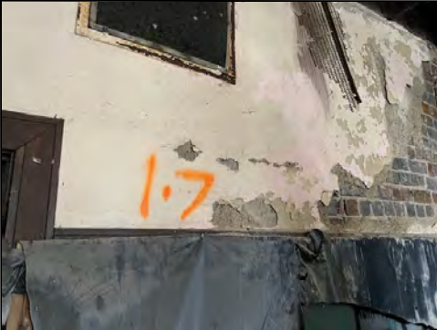
Sample 1-7, Plaster/Skim Coat-Walls
