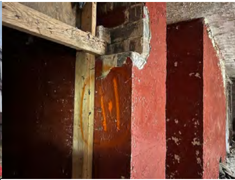
Sample 1-1, Plaster/Skim Coat-Walls
