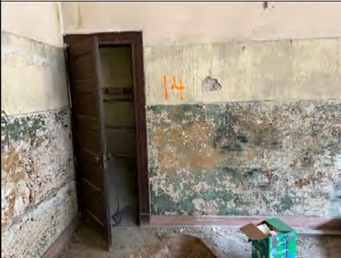
Sample 1-1, Plaster/Skim Coat-Walls
