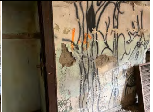
Sample 1-5, Plaster/Skim Coat-Walls
